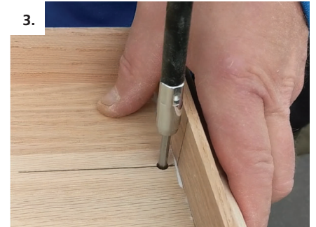
3. Glue and assemble nosing to tread with Clamex P-14 by engaging cam lock
