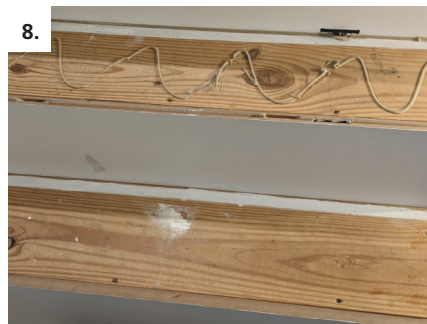
8. Install Tenso connectors and apply PL adhesive to rough framing and underside of tread
