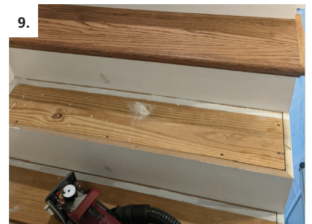
9. Tread is glued securely with no visible fasteners
